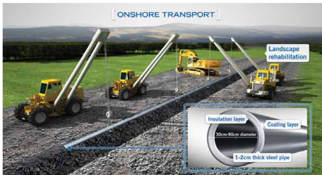
FIGURE 6.3 Onshore CO 2 transportation – pipeline construction
